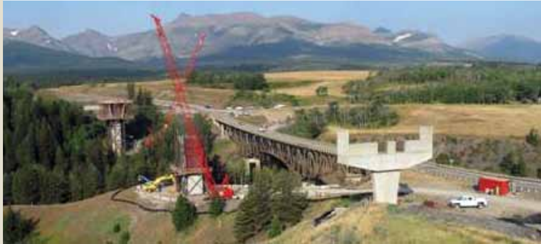
Bridge construction on U.S. Highway 2, spanning Two Medicine River.
