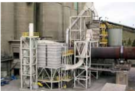
Montana City plant
